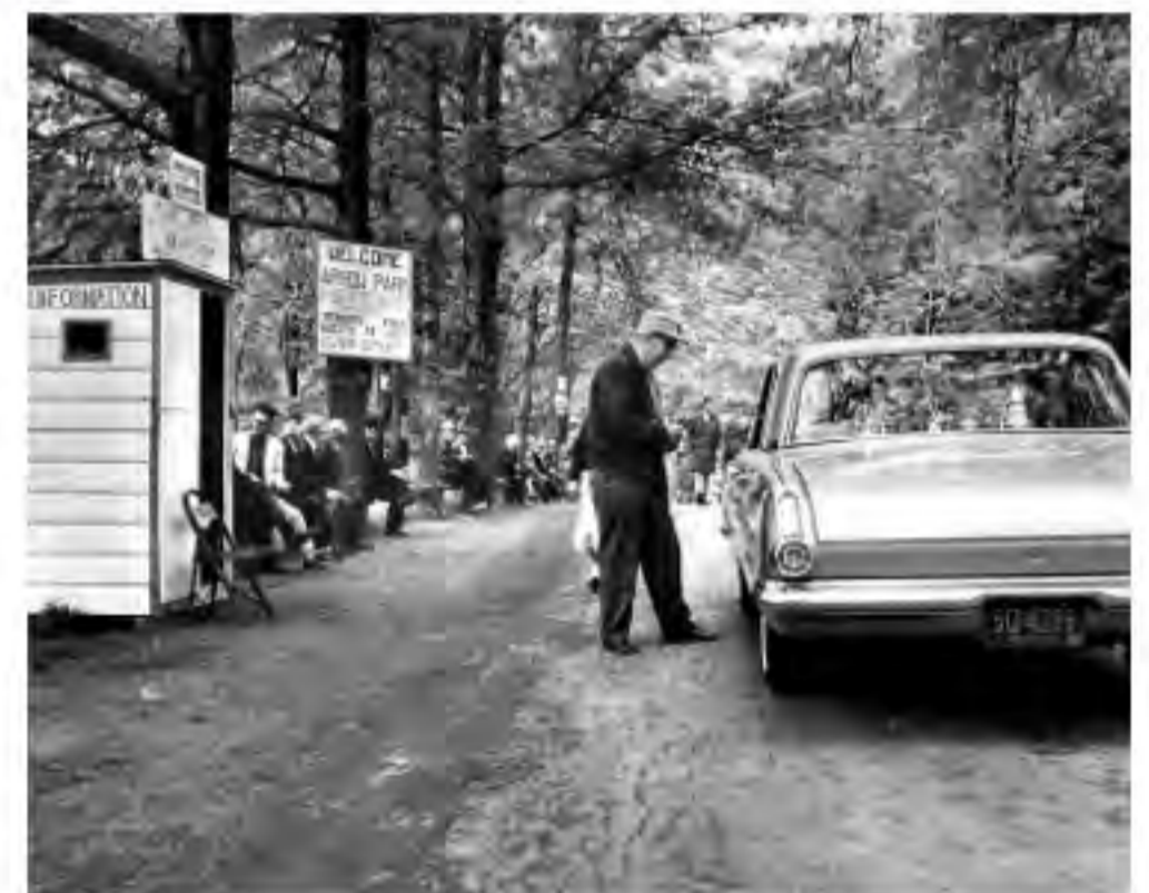
Top, the lodge originally was built in 1909 by Schuyler Schieffelin and his wife, Julia Cooper. The style of the home was progressive for its time and reflected the arts-and-crafts movement. Above, Harry the Clown at Arrow Park in the mid-1960s. Photo courtesy the Tomczak family.
