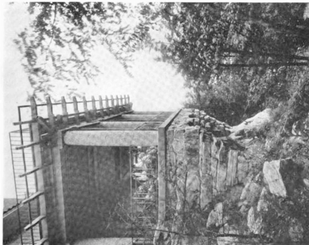
SUN PARLOR—HOUSE OF SCHUYLER SCHIEFFELIN, ESQ., MONROE, N. Y. Bowen Bancroft Smith, Architect.
